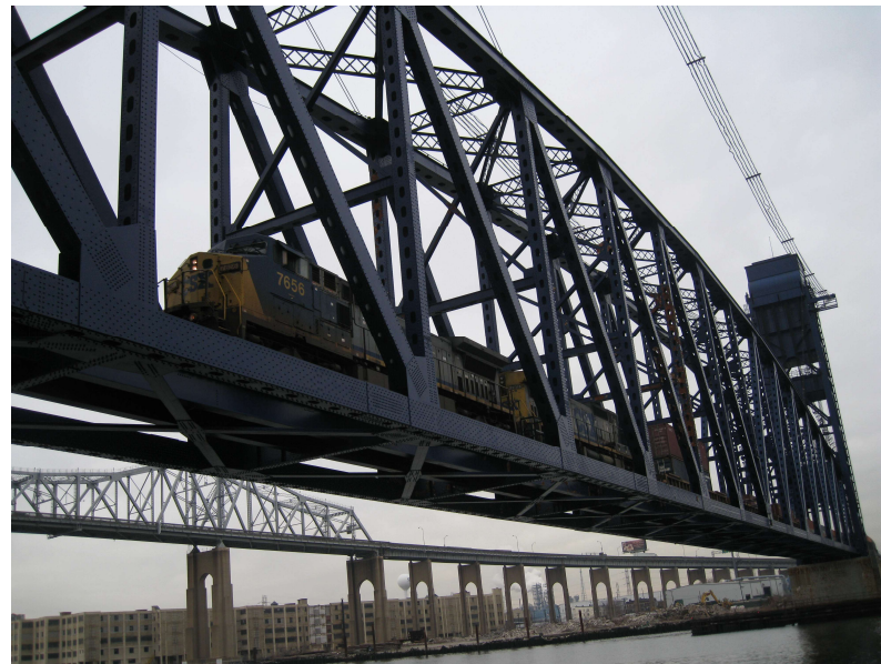
Arthur Kill Lift Bridge Tracks. Photo Source: NYCEDC
