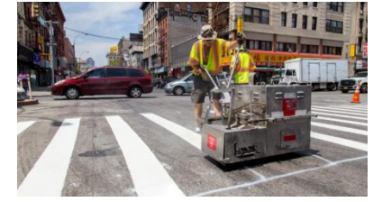
200M linear ft. of markings
